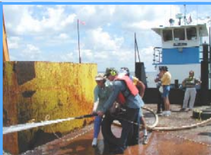
Controlling the high pressure hose.
