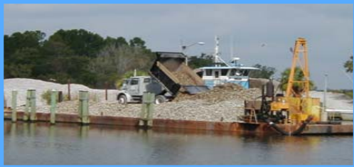
Loading the barge with cultch material.
